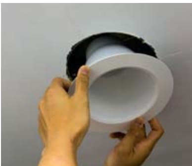
Installation of a downlight
